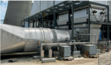
John E. Amos Power Plant, Unit 3, West Virginia, USA, 2006-2007. 1300 MW(e) boiler. 2 stage fan with nodular cast iron blades
