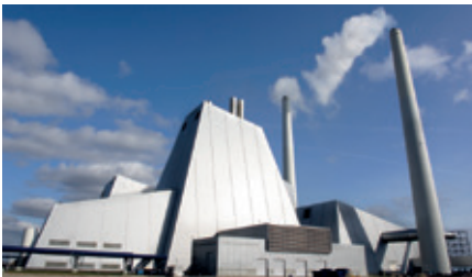
Power Station Avedøreværket, Denmark 2002. 580 MW(e) boiler. 2 stage fan with aluminium blades
