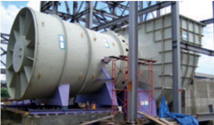
Uong Bi Power Plant, Vietnam 2004. 300 MW(e) boiler. 1 stage fan with nodular cast iron blades
