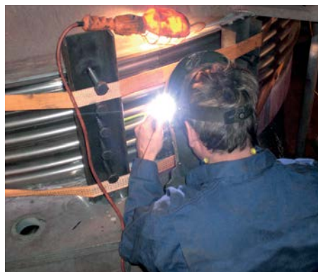
Installation of a clamshell metal expansion joint.
