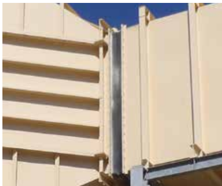
Acouseal installed in gas turbine air inlet.
