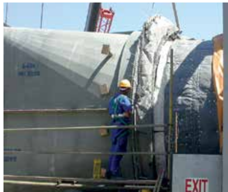
Installation of fabric expansion joint between the diffuser and diverter in a gas turbine system.
