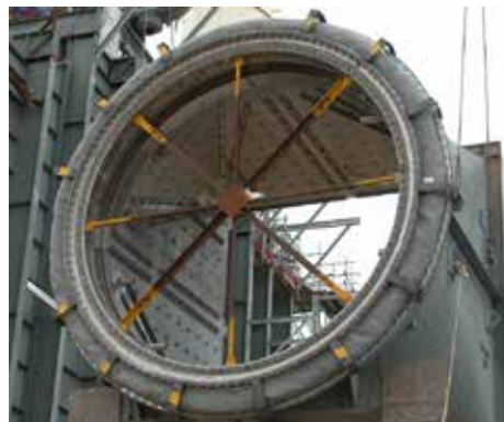
Installation of Combine-X on diffuser.
