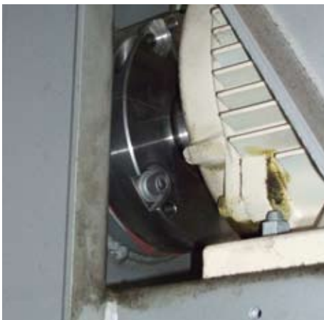
Espey™ WDKS-Eco, installed on a fan shaft Photo by courtesy of Aurubis AG
